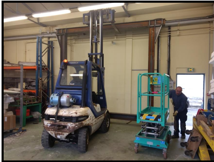
Figure 7-9. Installation of the long-term creep frame.
