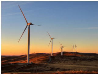
(c) Wind turbines
