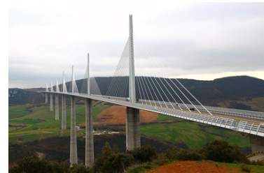
(e) Long-span bridges
