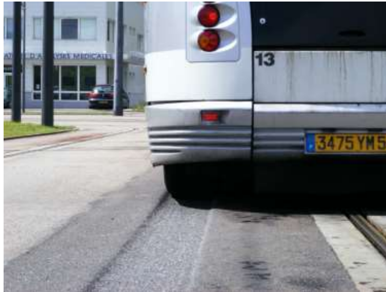
Figure 2-8 Example of rutting by a trolleybus ( http://transporturbain.canalblog.com/ 2019)
