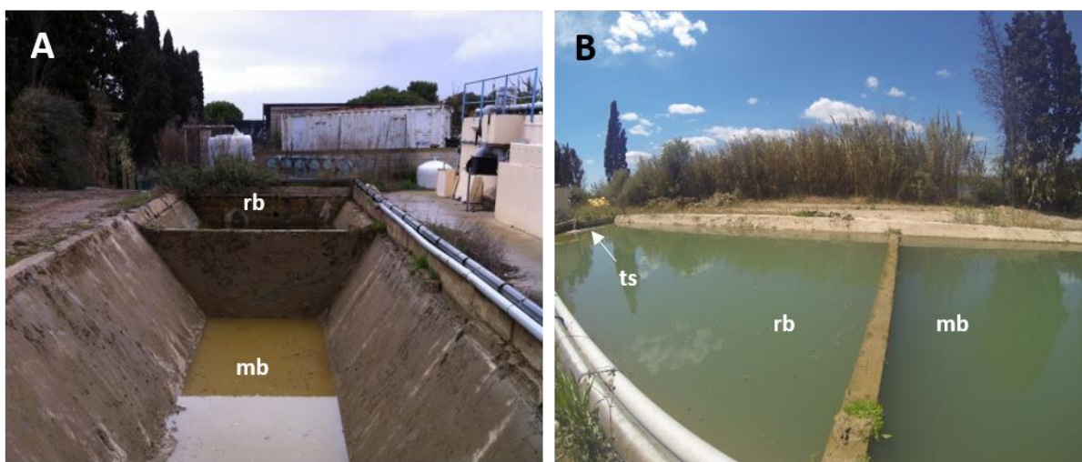
Figure 1. Retention basin of the Thermes de Balaruc-Les-Bains. Views of the mud maturation basin (mb), the water retention basin (rb) and the thermal spring water supply (ts) on February 28th, 2014 (A) and on May 12th, 2014 (B).
