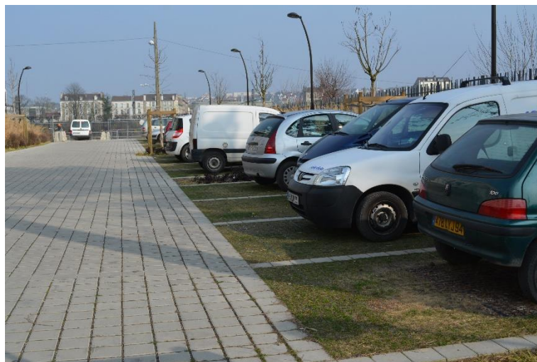
Figure II.16: Parking perméable de Villeneuve-le-Roi
