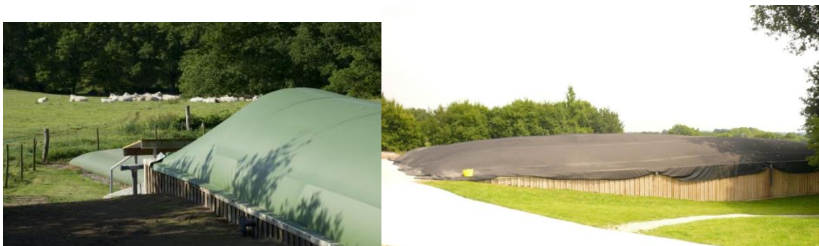
Figure 13 : GAEC du Bois Joly (sources : ARIA Energies, APESA)
