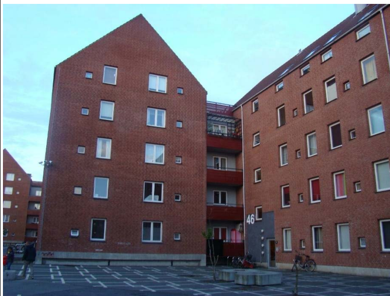
Figure 3.81 Low-rise marginalized social housing neighborhood in Nørrebro, Copenhagen. (Photo APLP, 20/05/2015)
