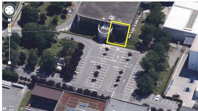
Figure 1.4.: HBS-Technal Headquarters – Toulouse (Google Maps)
