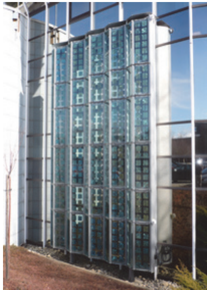
(a) Solar Modules on the Vertical Facade
