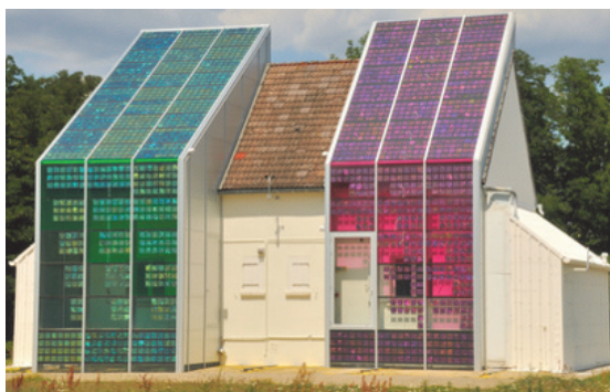
Figure 1.3.: ETNA Building – EDF R&D – Moret-sur-Loing
