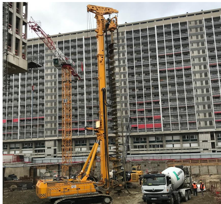
Figure 2.22 The drilling machine used to execute the piles
