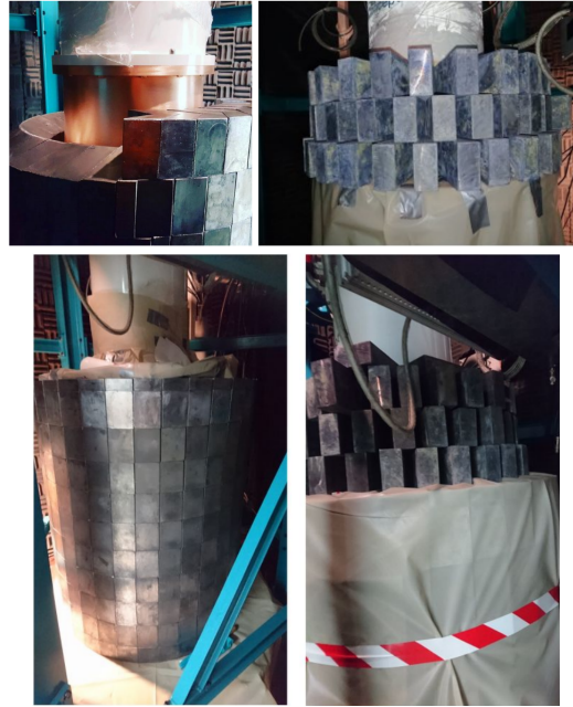
FIGURE 5.8: Lead shielding stages. Up left : the first 15 cm of lead installed in April 2019 (Stage I). Up right : 25 cm of temporary shielding above the 15 cm in June 2019 (Stage II). Bottom : Complete lead shielding in July 2019 with 25 cm of lead bricks above (Stage III).
