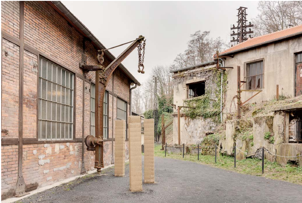
Supports, in situ
