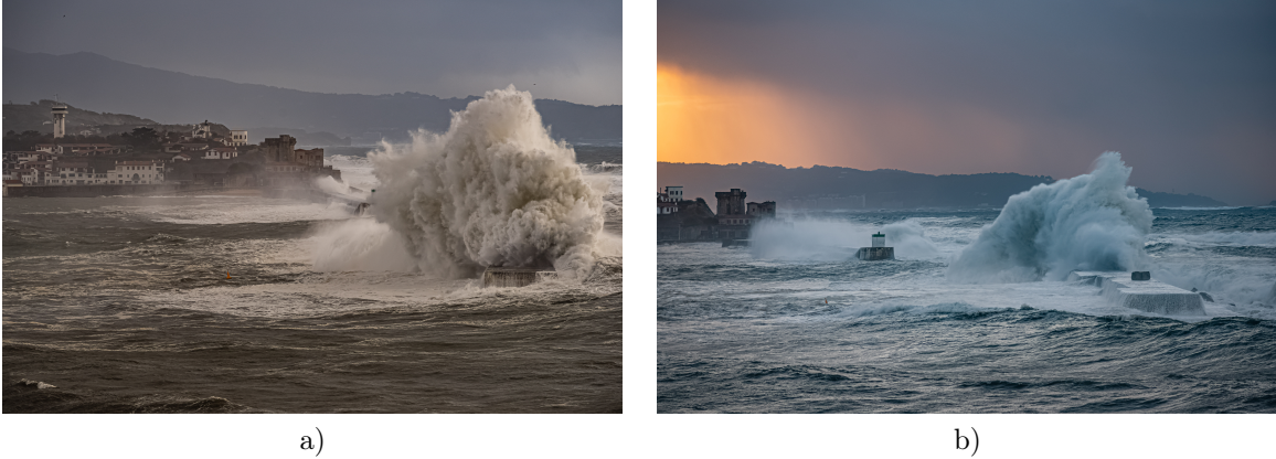
Figure 2: Snapshots from the storm of February 28, 2017. a) photograph of a wave impacting the Artha breakwater, b) photograph of a 50T block displaced by a wave during this storm.
