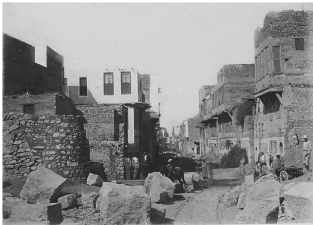
Figure 1.1.17. Percement de la rue Clot-Bey.
