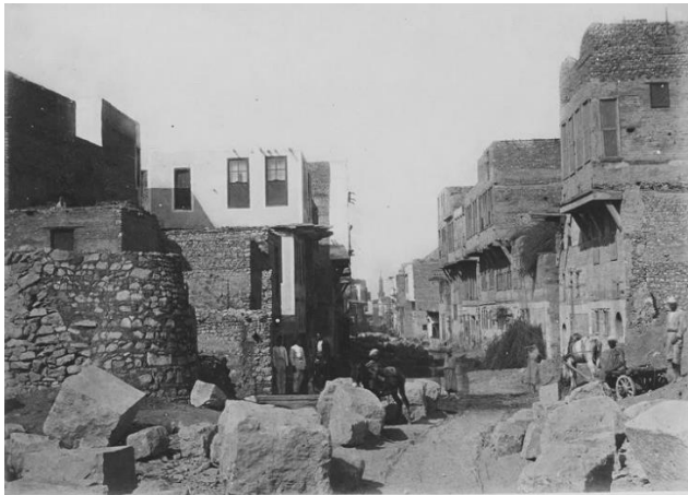
Figure 1.1.17. Percement de la rue Clot-Bey.
