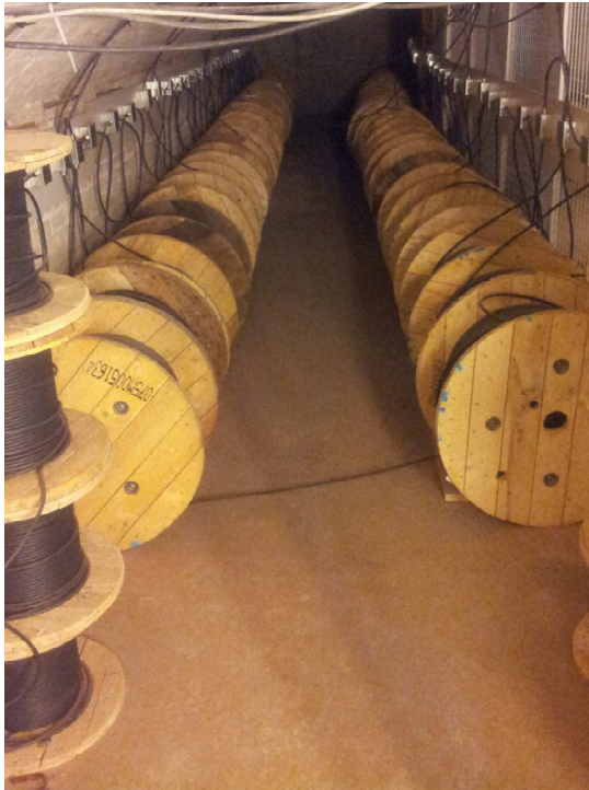
(a) Arrangement of cable drums
