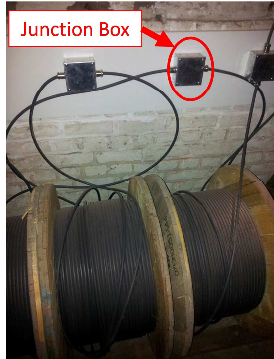
(b) Junction between two cable sections
