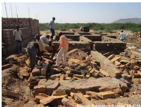
Image 34. Demolition of houses' plinth because of improper execution (left).
