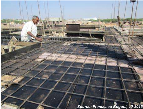
Image 8. A contractor fixing the centering before casting the roof slab (left).
