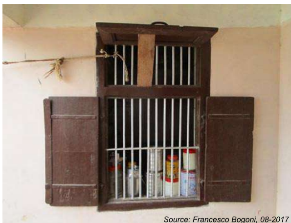
Image 36. A window reemployed from demolished houses (left).
