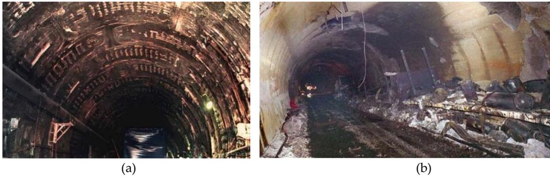
**Figure 3.17** After fire: a) tunnel under La Manche in 1996 [32], b) tunnel Mont Blanc [33].
