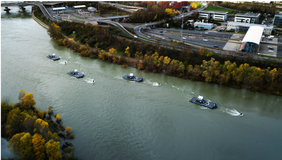
Fig. 1.6: Four hydrokinetic vertical turbines in the Rhone (HydroQuest).
