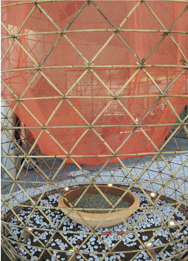
Figure 8. Prototype of the vase-shaped Warka Water version 1, showing a bamboo structure supporting a single layer of Raschel mesh (orange), as presented at MAXXI (national museum of contemporary art and architecture) in Rome, Italy in 2014. © Ana Rewakowicz, 2014.
