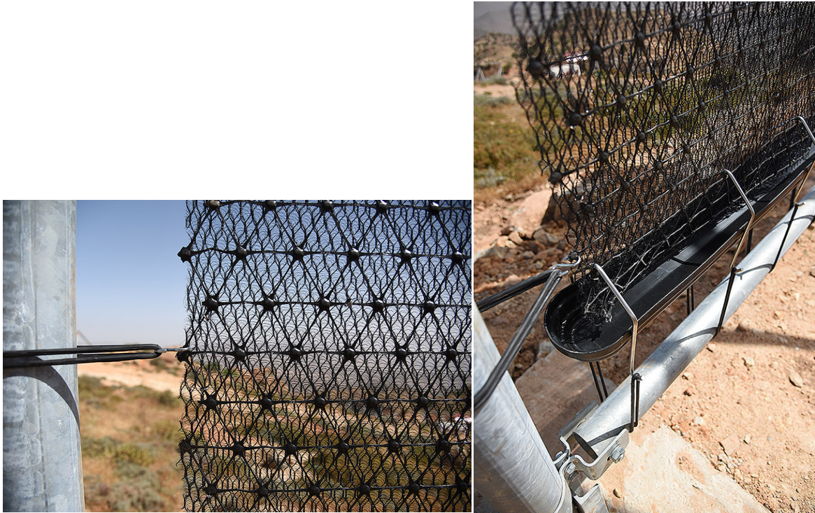
Figure 6. Details of the CloudFisher™ system installed on Mount Boutmezguida, Morocco. Left image, a sturdy plastic grid (large equilateral triangles) is visible on leeward side with diamond/hexagonal mesh (thinner smaller fibres) visible behind the plastic grid. One of the rubber expanders can be seen connecting the plastic grid to the steel frame (vertical structure at left edge of photo). Right image, rubber bands support a collecting gutter (black) between the plastic grid and the steel frame. © Ana Rewakowicz, 2017.
