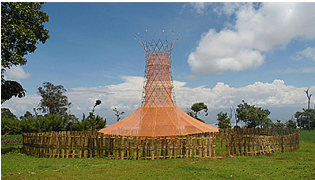
Figure 9. Prototype of a tower-shaped Warka Water version 2. © Arturo Vittori, accessed from https://lightroom.adobe.com/gallery/3040b751460a4b70bc4c79179dd1c018/albums/889f0b27c0da4833abfd4409b5532f10/assets/f67e6caf28236b5018a66b90d2a233dd .
