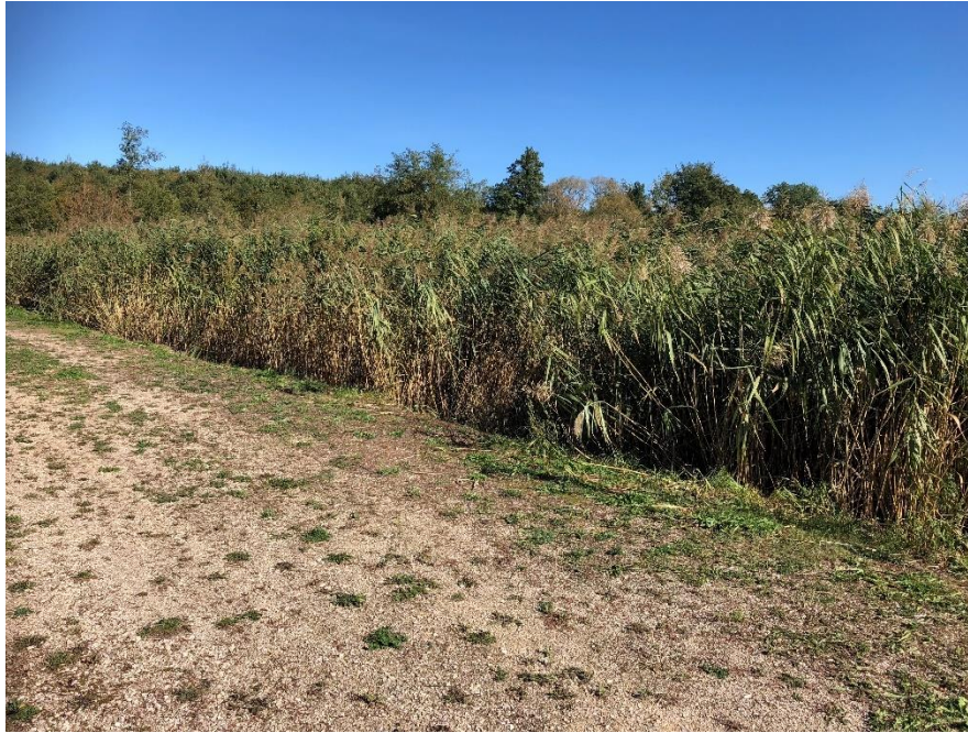
Figure 19: Bed filter planted with reeds from the 2 nd stage Constructed wetland in Falkwiller (Grand Est, France).
