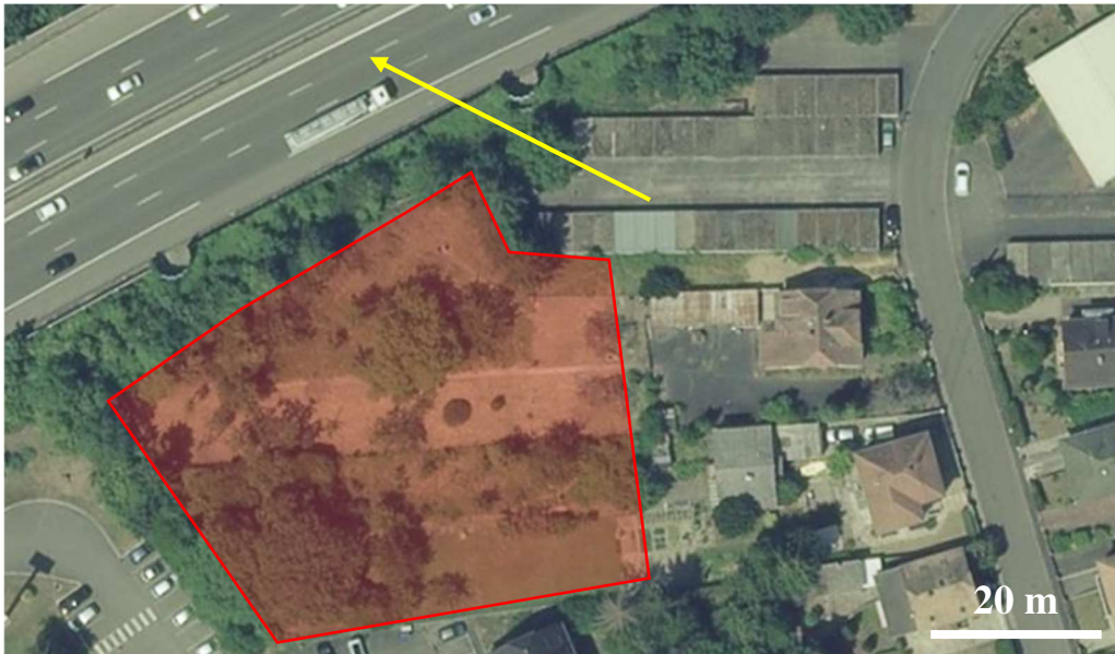
Figure 8.2 – Satellite image of Ostwald with the area studied (in red) and the highway (yellow arrow).
