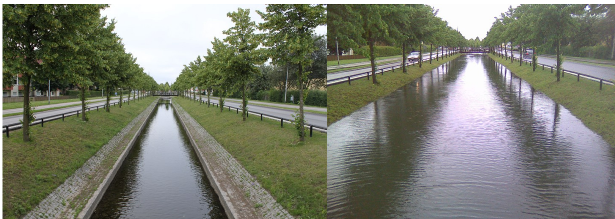
Figure 42 The Linnaeus Canal, functioning as a storm water container, before and after a rainfall event. Source: EEA, 2016b.
