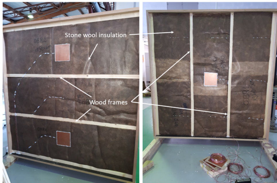
Figure 5.6: Tested WFW wall: (left) Rear and (right) front views of the insulation layer of the wall.
