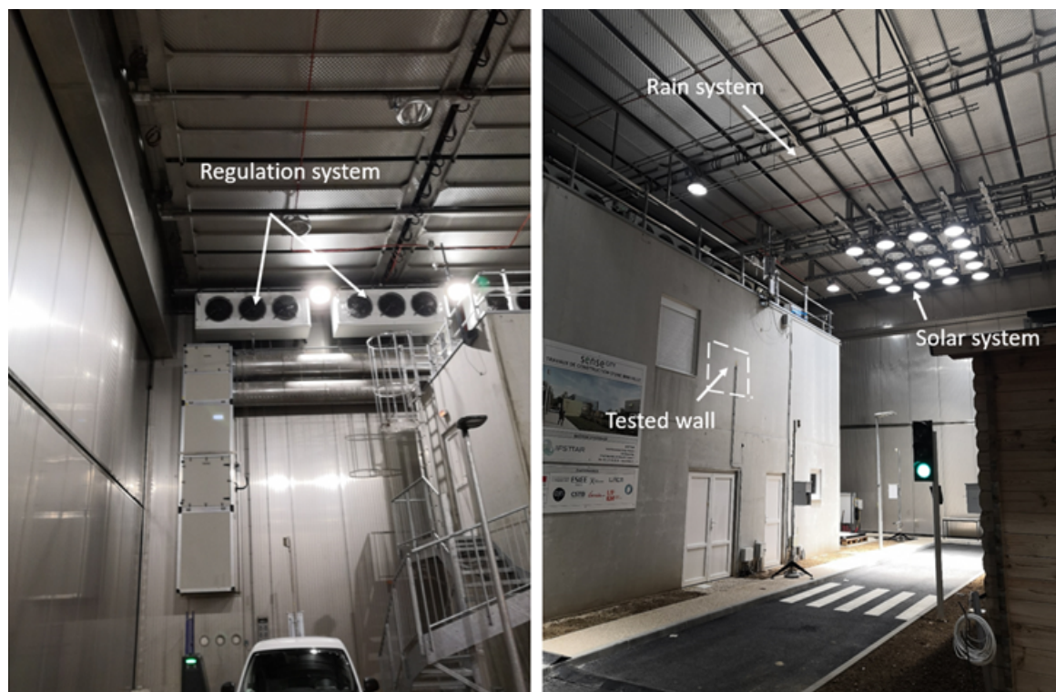
Figure 5.16: Regulation systems used in the climatic chamber Sense-City.
