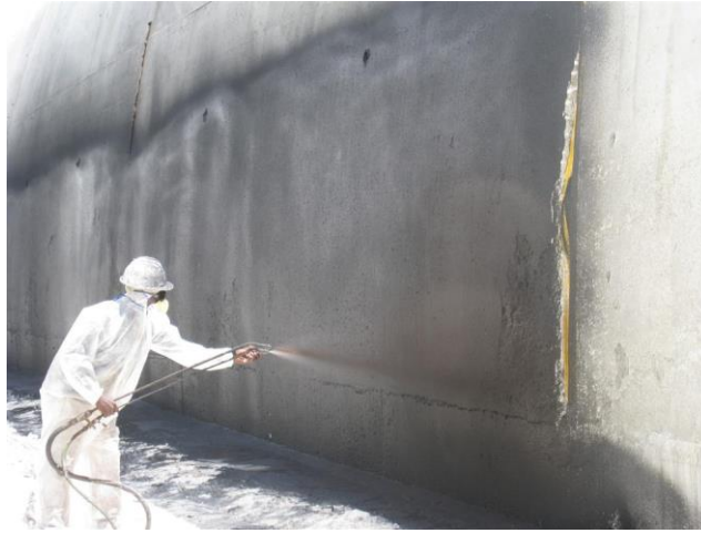
Figure 90 : External waterproofing coating
