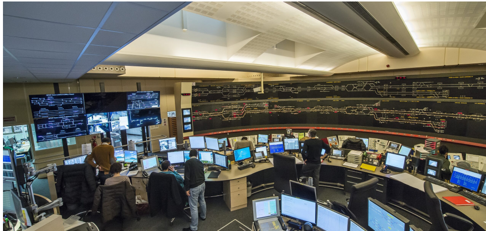
Figure 1.3.: Control center of the commuter train line 'RER B' of Paris
