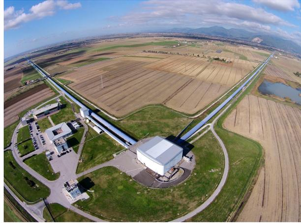
**Figure 1.9:** Aerial view of the Advanced Virgo detector. The two 3 km arms of the interferometer meet in the central building where the laser beam is generated, and five mirrors, including the BS, are hosted. Optical benches used to acquire the interference pattern are also hosted in this building. On the left part, the other buildings host the European Gravitational wave Observatory (Italy) (EGO) offices.
