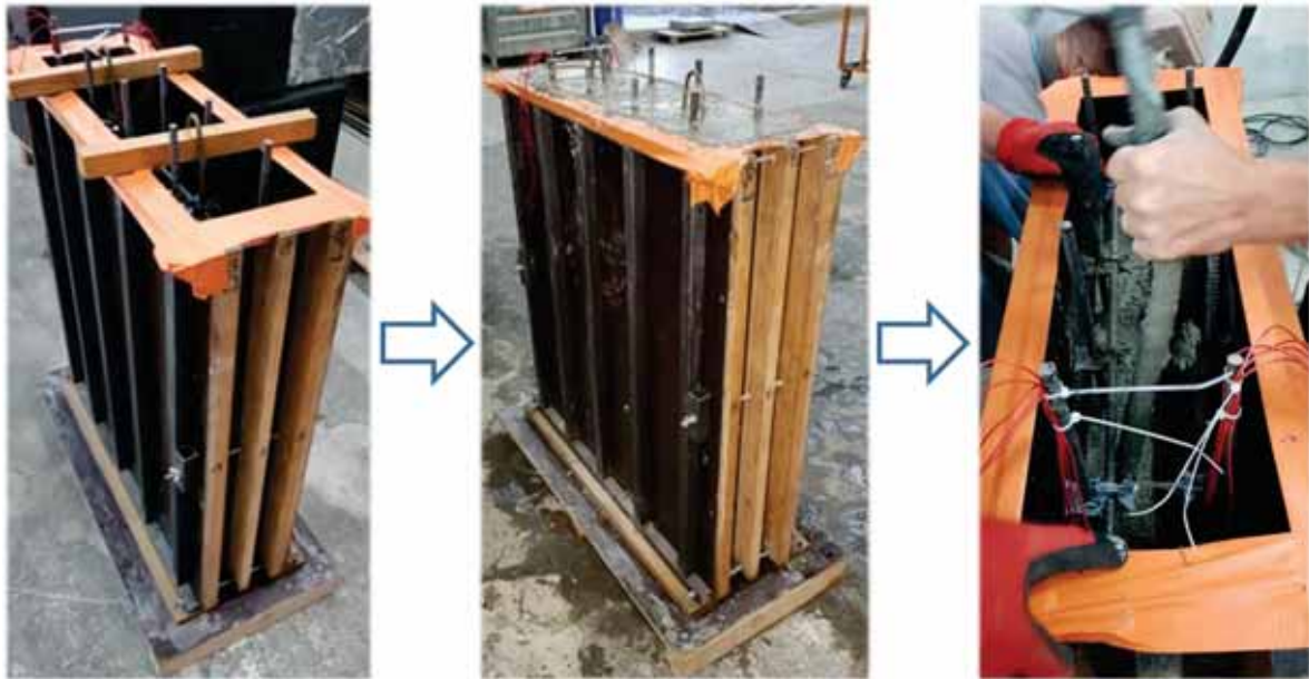
Fig. 13. Formwork and casting of the wall
