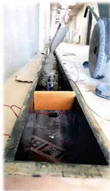
Fig. 17. Casting of the beam
