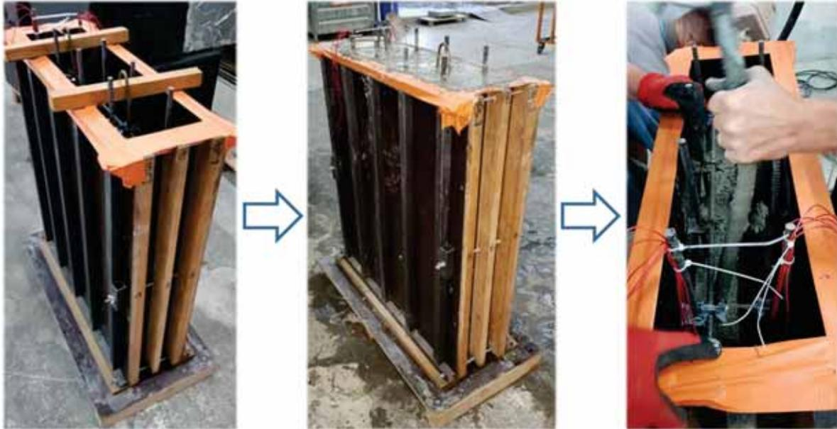
Fig. 13. Formwork and casting of the wall
