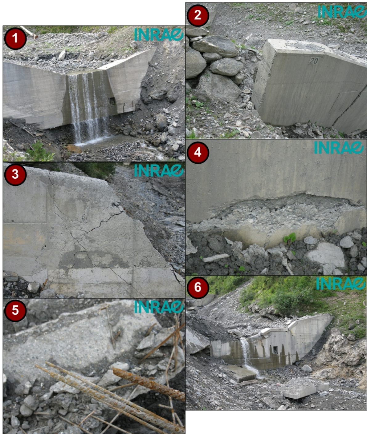
Figure 1.17: Examples on the types of functional and structural failures check dams may be subjected to: (1) scouring under dam's foundation; (2) erosion of banks due to lateral bypass; (3) presence of cracks; (4) concrete corrosion; (5) steel corrosion; (6) total destruction. Saint Antoine torrent, France, 2014. Source: ©INRAE/ETNA.
