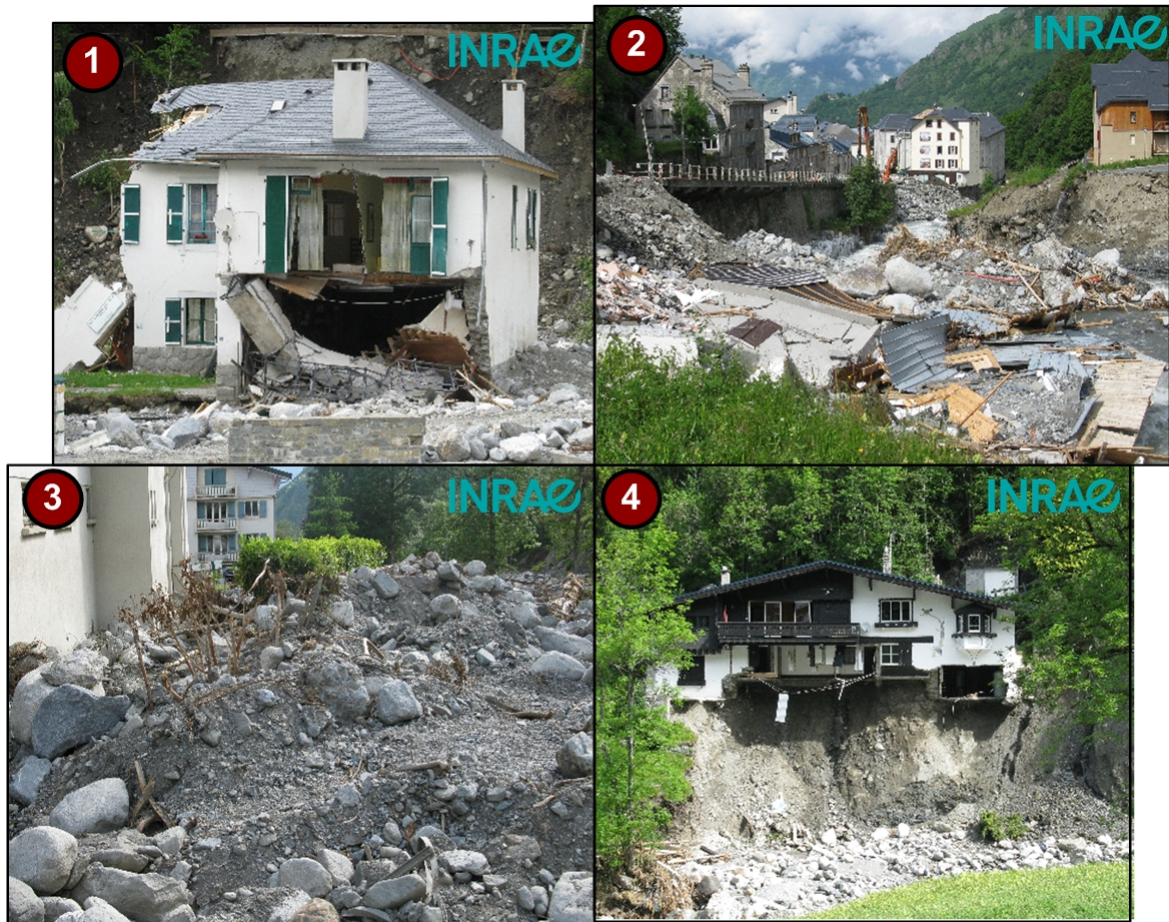
Figure 1.5: Damages resulted after torrential flood in Bastan à Barèges (Hautes-Pyrénées) , June 18, 2013. (1) and (2) destruction; (3) deposition; (4) scouring. Source: ©INRAE/ETNA.
