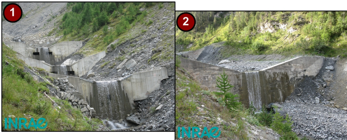
Figure 1.11: Torrent check dams: (a) Check dams series; (b) Single check dam. Saint Antoine torrent, France, 2014. Source: ©INRAE/ETNA.
