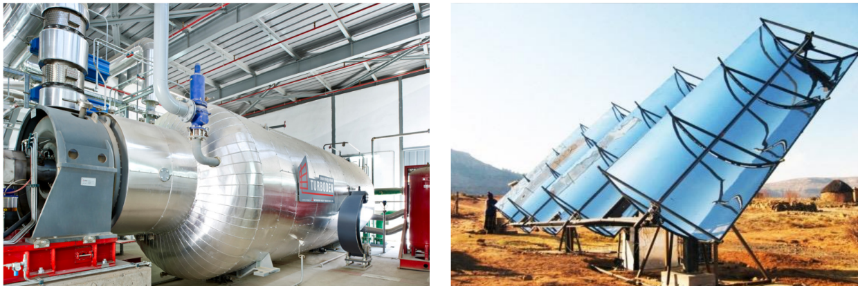
Figure 1.1: Examples of ORC units: (left) 2 MW Turboden ORC unit using heat recovery in a cement plant and solar thermal energy (Source: Colonna et al. (2015)); (right) Solar ORC unit installed in Lesotho (Africa) to help local people becoming electrically self-sufficient (Source: STG international).
