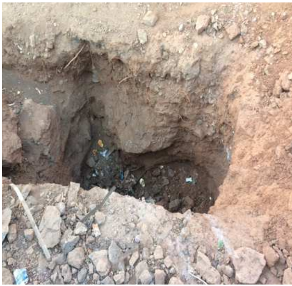
Example of a Pit
