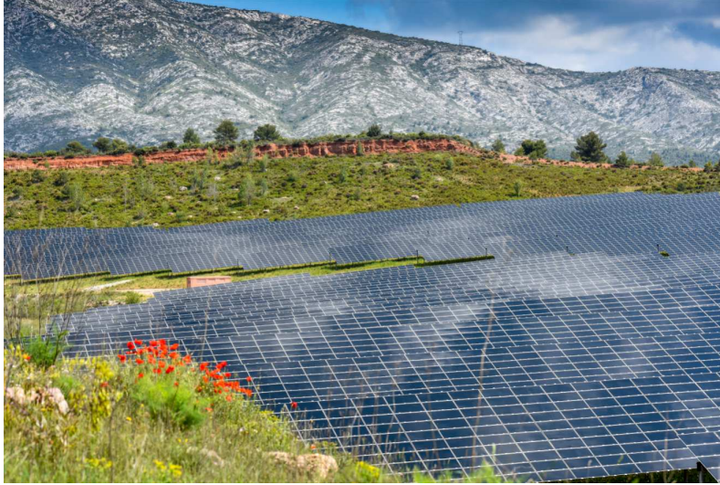
Figure 1.1: PV power plant from EDF Renewables installed in Puyloubier.
