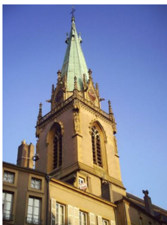
Figure 2. 3 : The bell tower of S. Martin's church with the original copper tiles before restauration.
