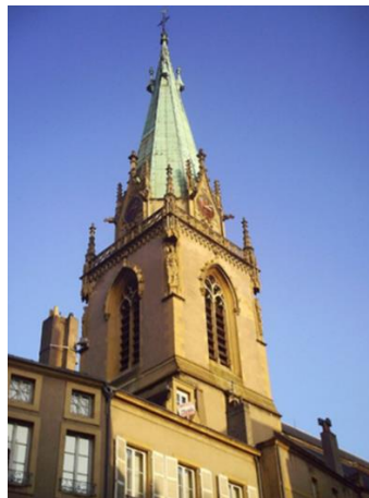
Figure 2. 3 : The bell tower of S. Martin's church with the original copper tiles before restauration.
