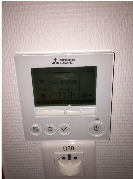
FIGURE 4.7: HMI installed in each room of the building.
