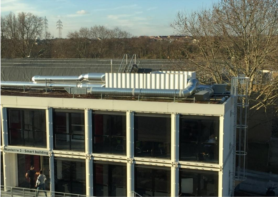
FIGURE 4.6: Installed weather station and VRF system heat pump setup on the building.
