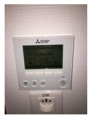
FIGURE 4.7: HMI installed in each room of the building.
