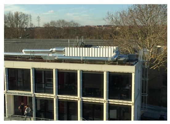
FIGURE 4.6: Installed weather station and VRF system heat pump setup on the building.
