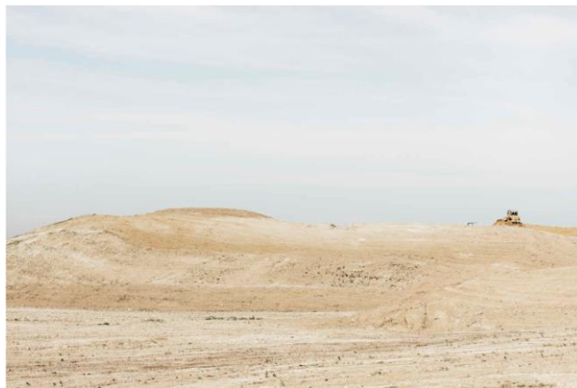
Figure 0.1. Inert waste storage quarry at Thivernal-Grignon – Yvelines (credit to Simon Schnepf and Morgane Renou [4])
