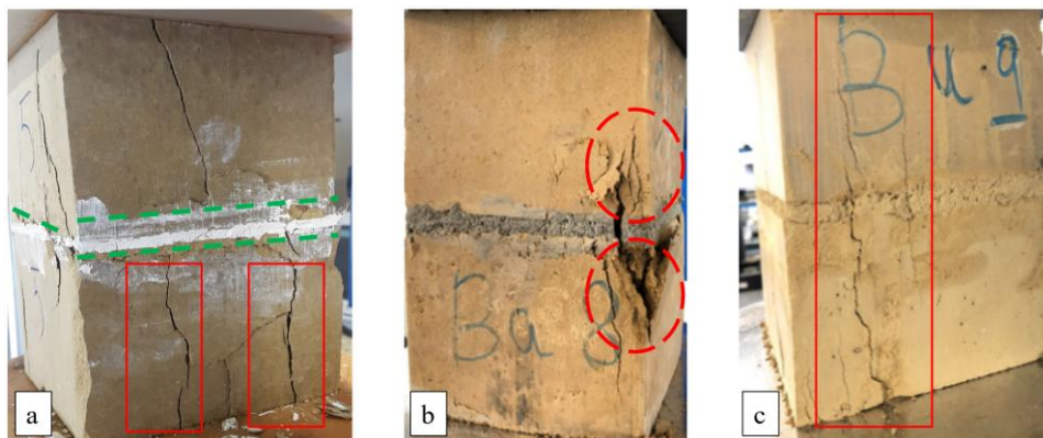
Figure 5.9. Examples of failure patterns of masonry; vertical cracks in the block then sliding at the interface (a); block crushing (b); vertical cracks (c)
