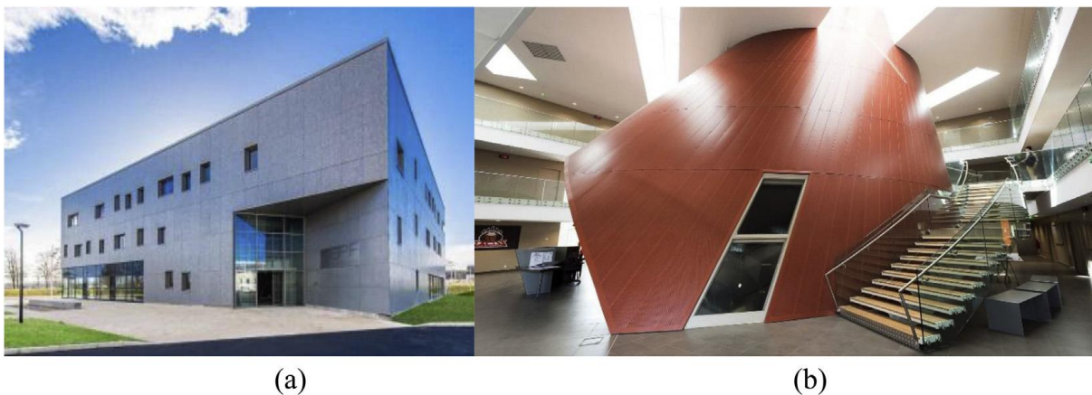
Figure 3-1 : EPF school building: (a) north-east view; (b) inside view.
