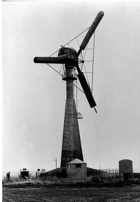
Figure 1.3: Gedser wind turbine, 200 kW,  $D = 24$  m, Denmark 1957 (Source: [5])
