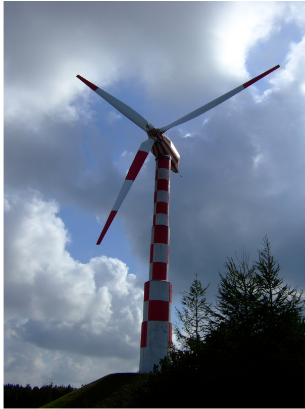
Figure 1.4: TVIND wind turbine, 2 MW, D = 54 m, Denmark 1977 (Source: [6])
