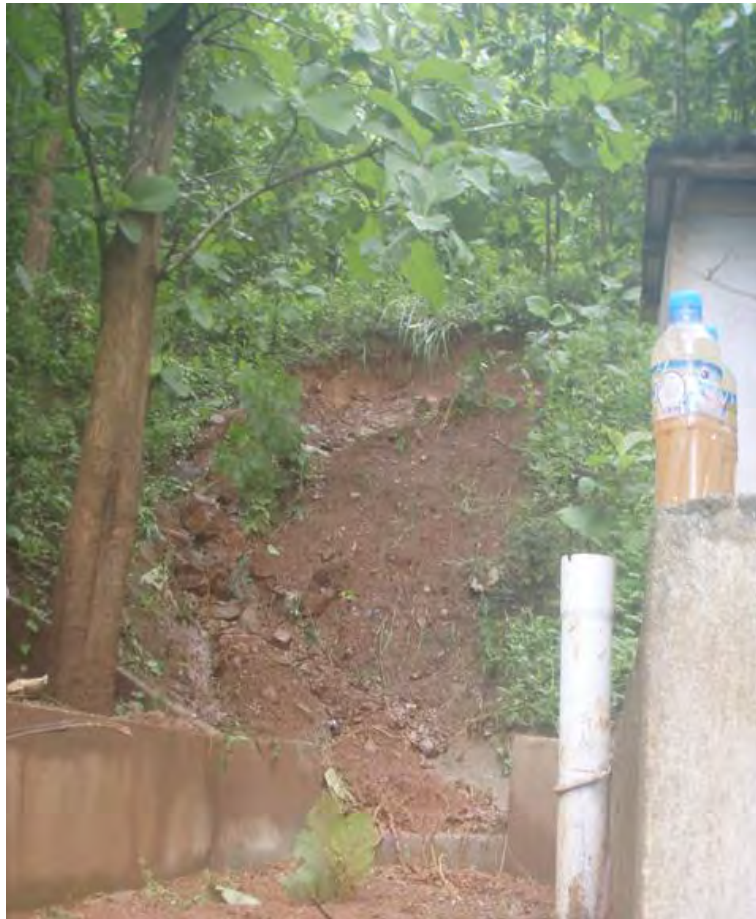
Figure 6.10: Landslide occurred behind the weir of S8 in the Houay Pano catchment
