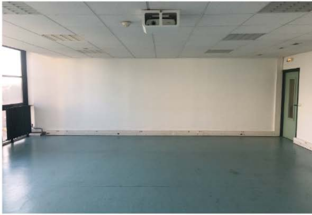
a) Front Wall
