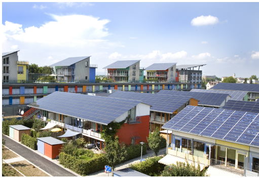
(a) Installed rooftop PV in Freiburg im Breisgau, Germany.
