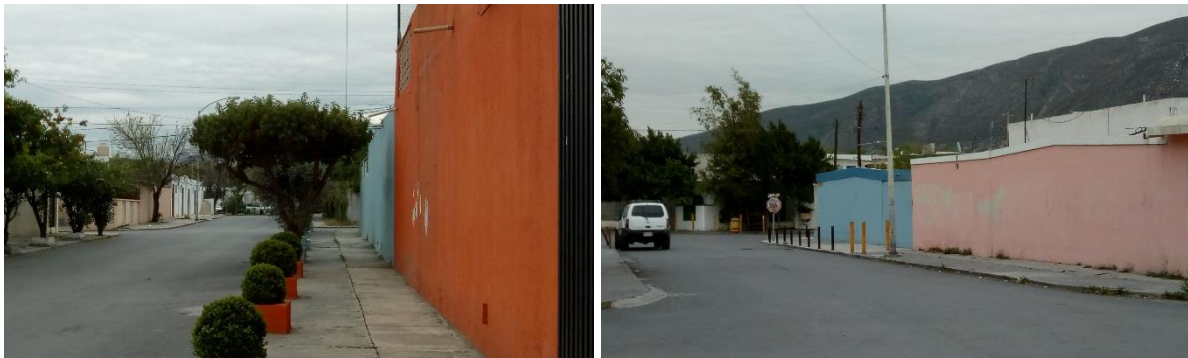
Figure 79 View of blocks of Loma Linda.
