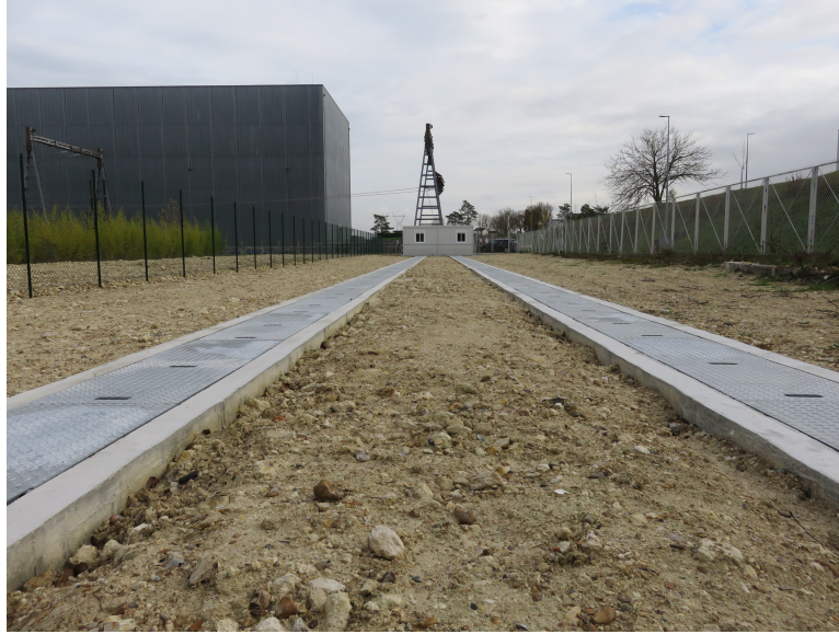
Figure 4-45: Reinforced concrete ducts covered by steel plates in the testing facility.
