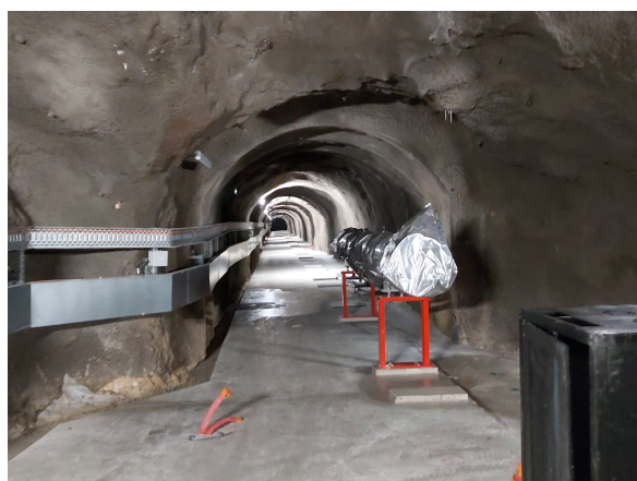
Figure 1.8 – The first section of the vacuum vessel bolted in the Miga gallery.
