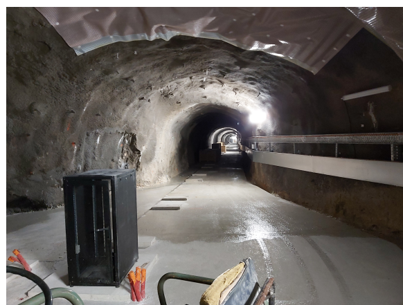
Figure 1.9 – View of the second orthogonal gallery.
