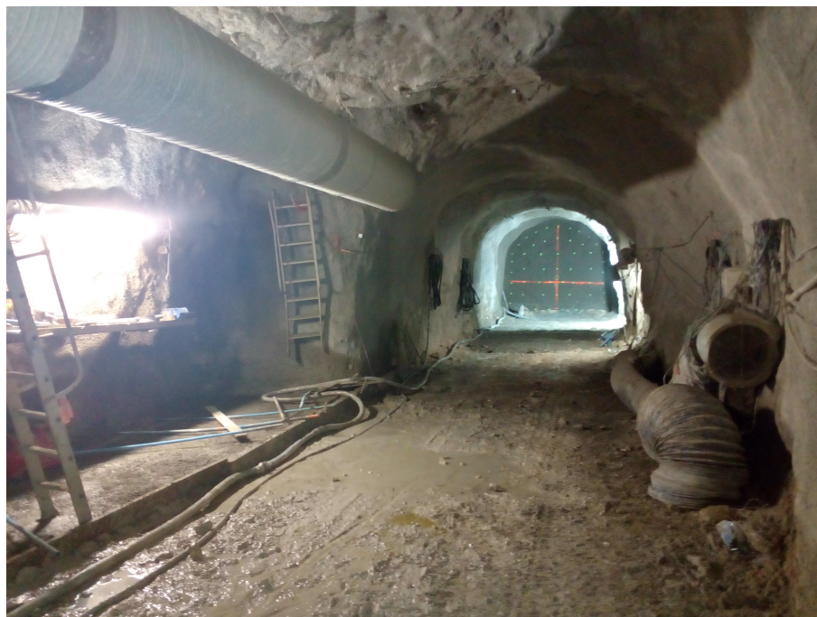
Figure 1.6 – Glimpse at the front of the gallery being drilled before blasting.
