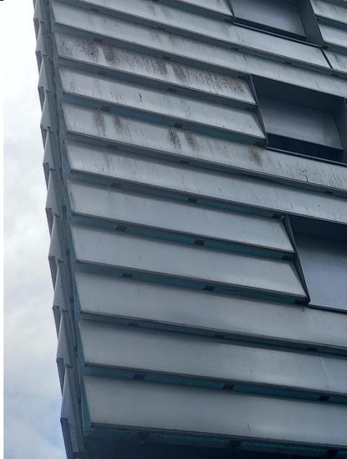
Figure 66 The inclined panels, spaced at approximately 150 mm intervals are attached to a concrete support insulated with several layers of insulation in order to reach the environmental objectives of the objectives of the project (Climate Plan of the City of Paris) and obtain the BBC label. *Source M. Apostolou*
