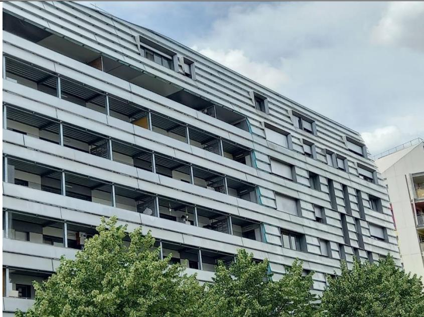
Figure 63 The main facade of the building is, in fact, a cladding in extruded polycarbonate, made with inclined panels arranged in tiles. Source M. Apostolou
