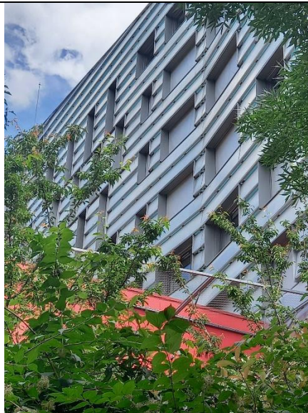
Figure 39 Building E1, View from the park. One can see the creche in red colour. The E1 building is developed mainly along the rue Cardinet, according to a succession of different opaque or glazed elements arranged according to a random rhythm, accentuated by the different colours of the elements characterizing the building's cladding. Source M. Apostolou
