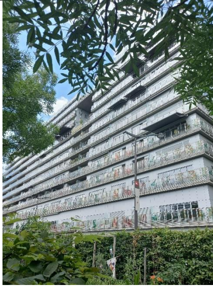
Figure 126 E5 building, south façade. Source M. Apostolou
