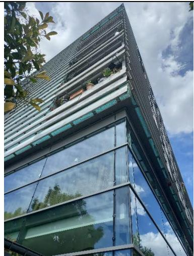
*Figure 40 The base of the building E1, which houses the shops and the crèche, is closed by a double height glass curtain wall. Source M. Apostolou*
