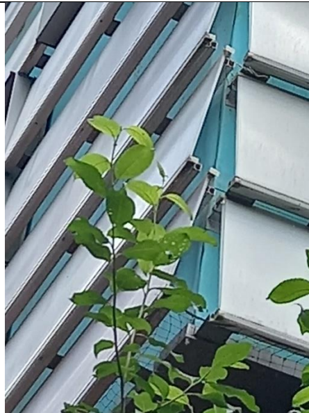
Figure 67 detail of the inclined panels of the façade of the E1 building. Source M. Apostolou
