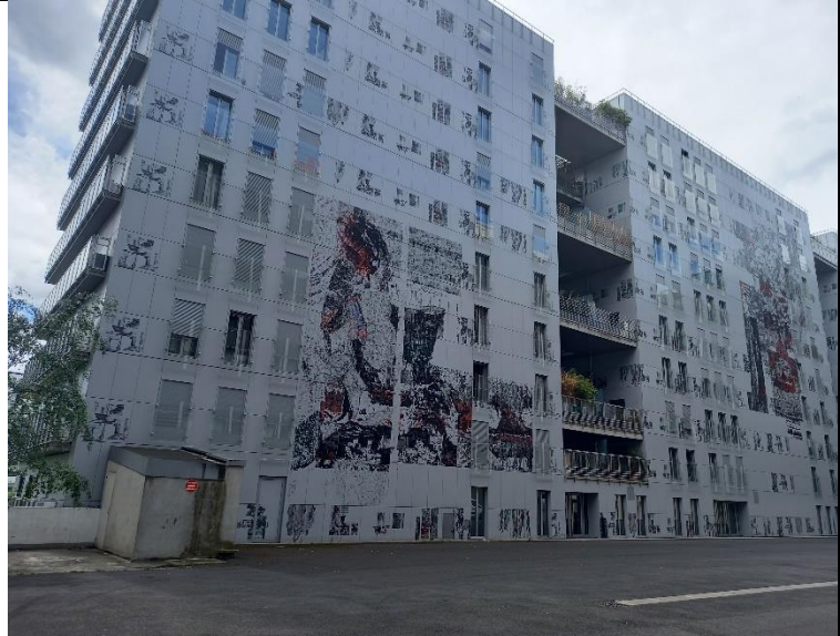
Figure 127 E5 building, north façade opposite to Ibis Hotel. Source M. Apostolou
