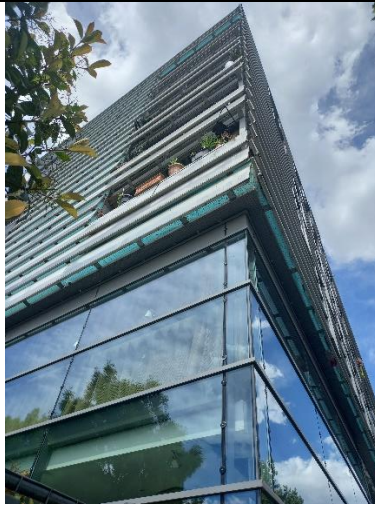
Figure 40 The base of the building E1, which houses the shops and the crèche, is closed by a double height glass curtain wall. Source M. Apostolou
