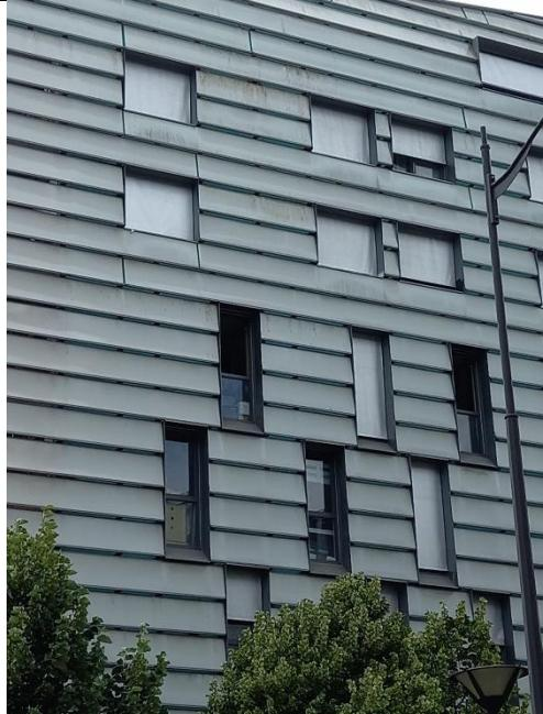
Figure 54 The glazed parts of the building are made up of mixed aluminium-wood joineries in double insulating glass. .
